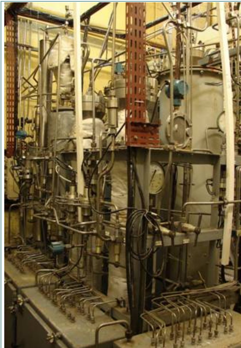
Picture. View of the plant in action
